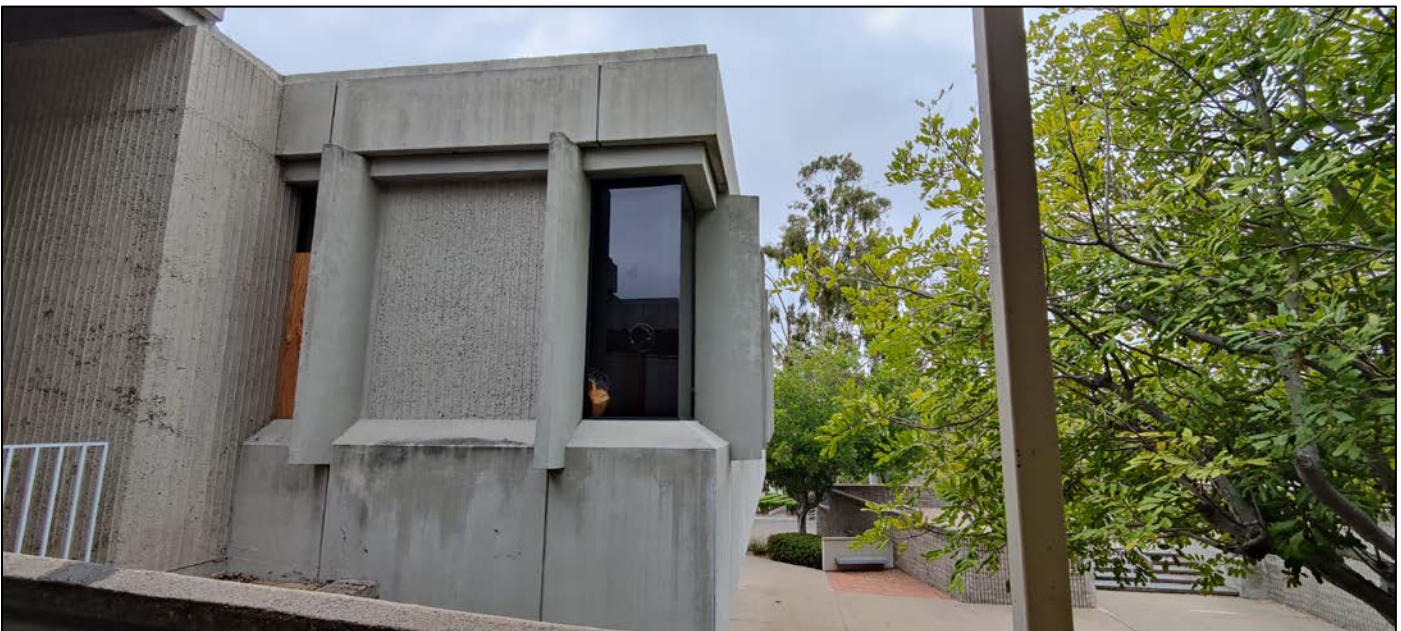
Second floor, southwest elevation, close-up of window configuration, facing east
