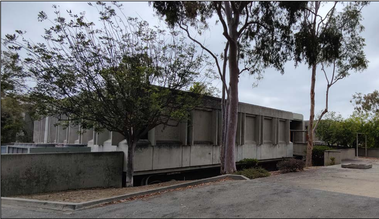
Oblique corner of northwest (left) and southwest (right) elevations, facing northeast
