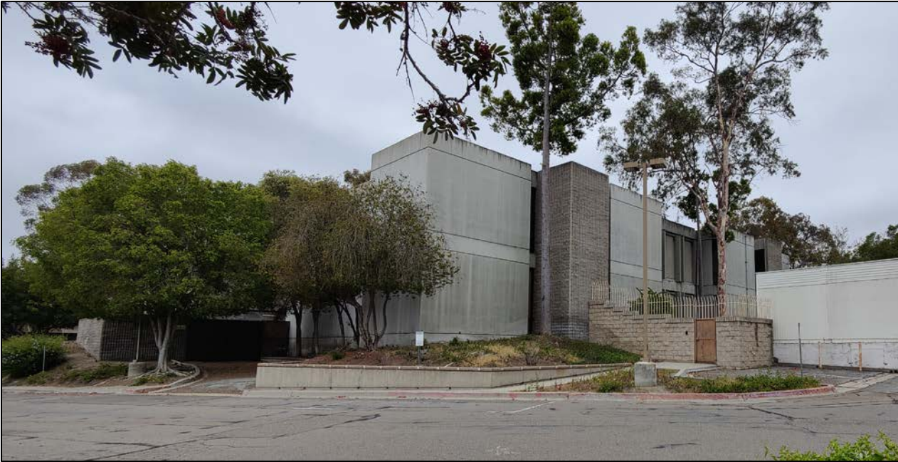
Oblique corner of southeast elevation (left) and northeast elevation (right), facing southwest
