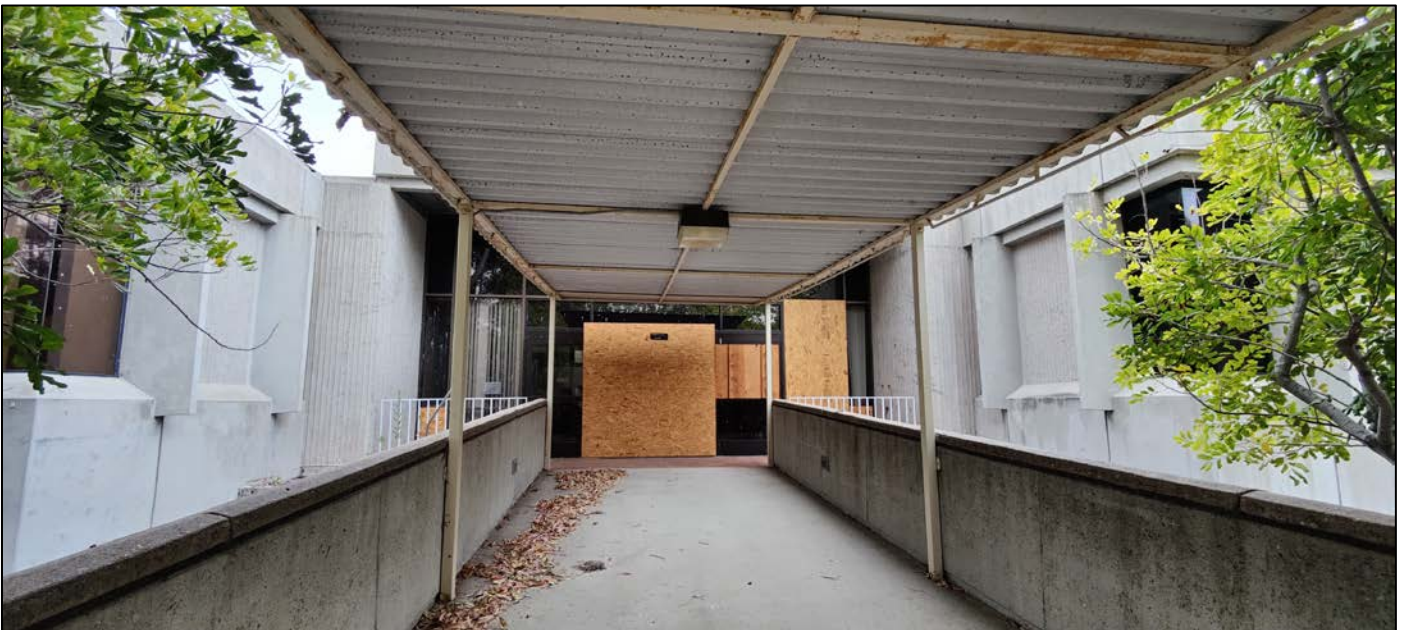
Primary entrance at second floor of southwest facade, facing northeast
